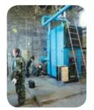
As a result of this effort, two AKM boilers working on wood waste and manufactured in the city of Tver were installed in the boiler plant. The boilers have rotary grates that direct hot air to sawdust drying, which allows using wood waste with high moisture content. The efficiency of the new equipment is 80%.
